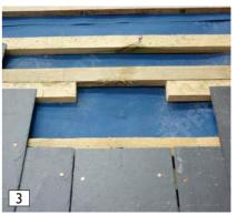
Fix an additional 1.2m support batten above the cut batten (spanning two rafters) and nail to the adjacent rafters.
