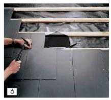
Fix the cut slates in position, leaving the underlay opening exposed.
