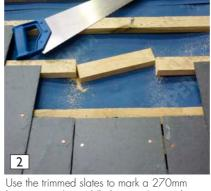
Use the trimmed slates to mark a 270mm long gap in the middle batten. Cut out this section of batten.
