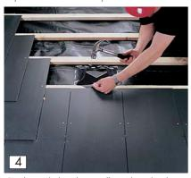
Cut the underlay diagonally and pin back onto the surrounding battens and rafters. For rigid sarking board, cut-out the rectangle.
