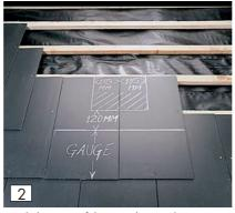
Mark the area of the two slates to be removed (hatched area shown above). Cut out this area.
