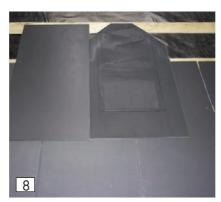
Fix the slates either side of the vent, ensuring that they overlap the side flashing by the correct distance. 600mm x 300mm slates should be aligned with the vertical weather bar (see guide marks on vent).
