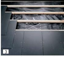
Using the cut slates as a template, mark the underlay diagonally as shown. This is the cutline.
