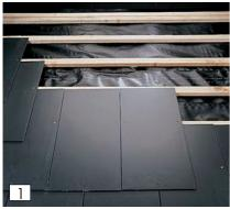
Decide in which course the vent is to be fitted and lay slates up to the course below. Lay the two slates directly below the vent.
