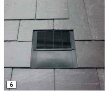
At gauges below 225mm, slight trimming of the slates in the course above the vent, may be required.
