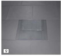
Continue to fix subsequent slate courses as normal. No slate cutting of the course above the vent is required.
