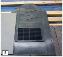
When fixing the adjacent 500mm x 250mm slates, they should abut the main vent body (see guide marks on vent).
