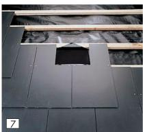
Slide the vent - spigot first - into the opening. Using the centring line on the vent, align with the joint line of the two slates directly below. Fix vent by nailing through centre nail holes.
